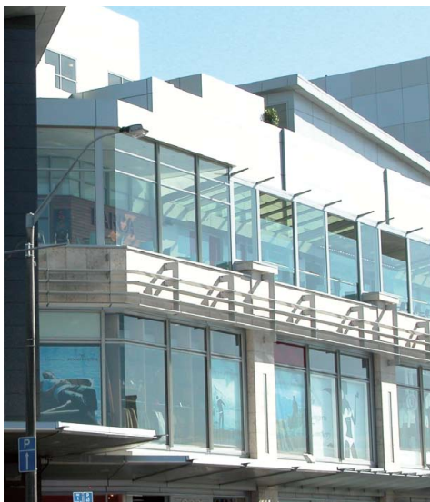
High level safety ventilation
